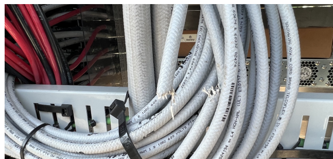
Left: Successful cuts and theft of wire in equipment cabinet. Top right: Cuts to wires on utility pole in conduit. Bottom right: Cuts to wires on utility pole in cabinet.
